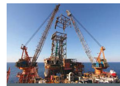
Specialist Maintenance Packages
